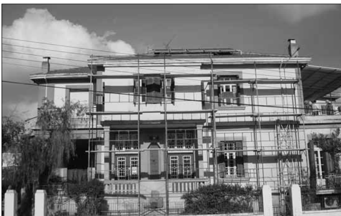
Before: Street Facade Scaffolded
