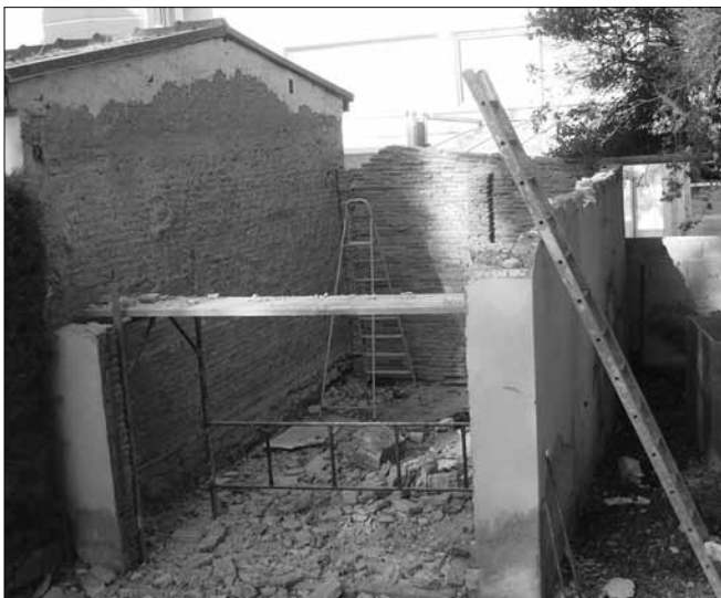
Before: CAARI Garage Being Re-Roofed
