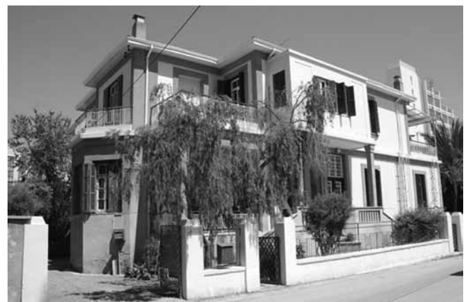
After: Street Facade Finished
